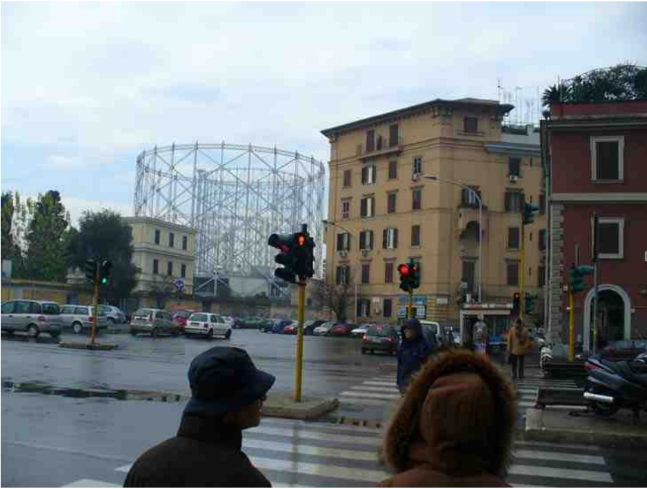
Intersection of Via del Commercio and Via Ostiense
