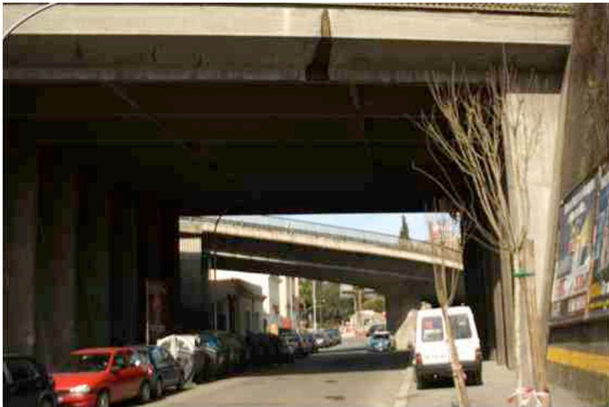
Figure 1.9 View of underpass of Corso di Francia (Shulman, 2009).
