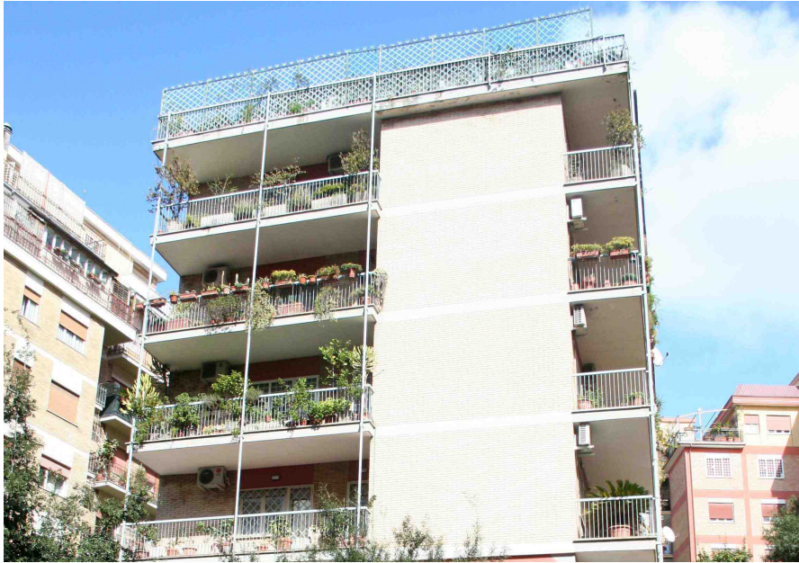
An example of the 6-7 Story Mixed-Use Residential Building located in southern Donna Olimpia.
