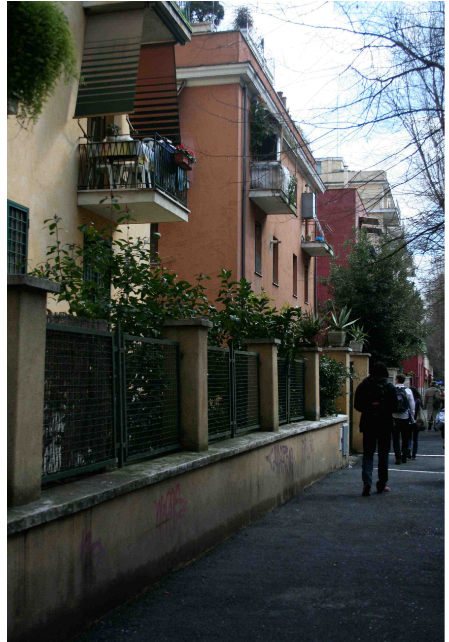
Type 1 5-6 Story Residential Apartment Buildings located in the northern part of Vida di Donna Olimpia
