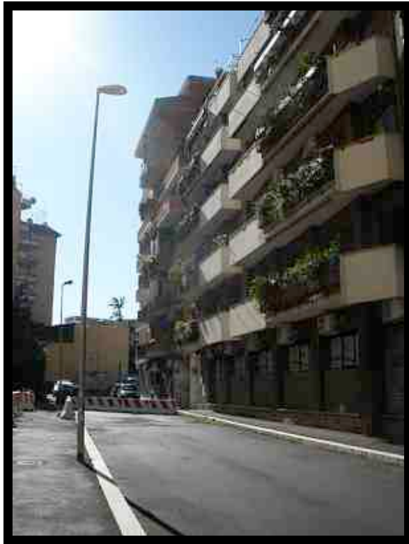
Blocked off portion of Via Asconio Pediano
