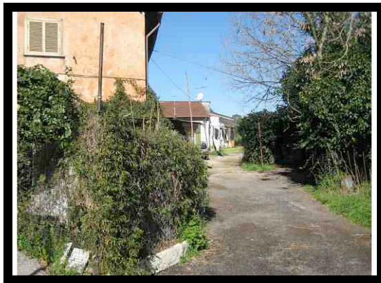
Houses in “Disconnected” Area
