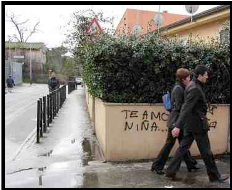
Retrofitted sidewalk on only one side of Via Cincinnato
