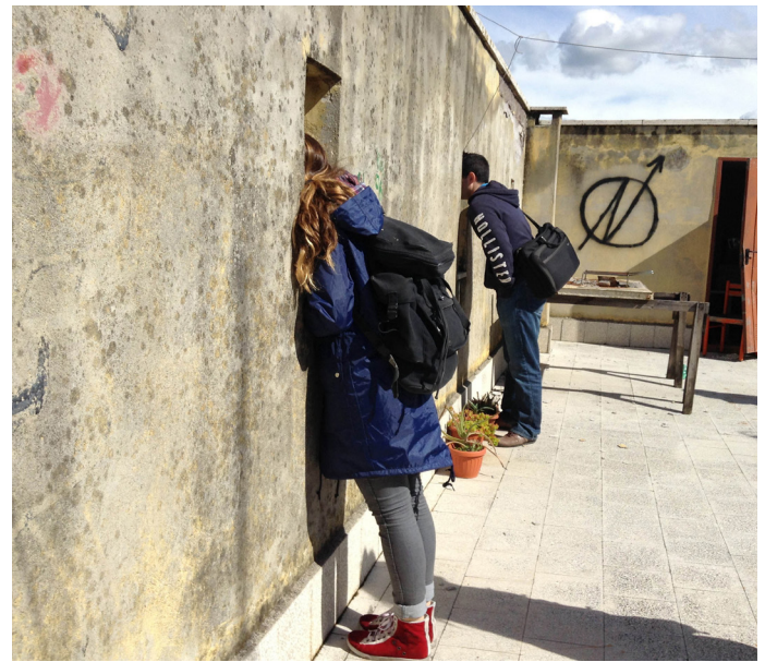
The Roof of La Talpa (Photo: Diana Folla)
