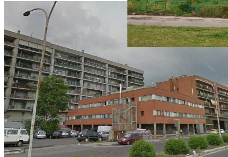
Figure 4.44. Informal Settlement in former office space
