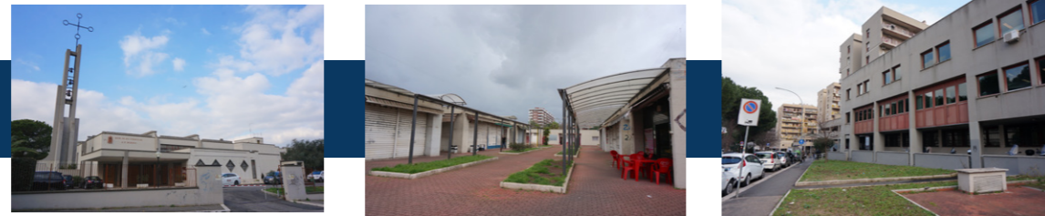
Figure 2.10. Public Building Photos (left to right: church, neighborhood market, employment center)
