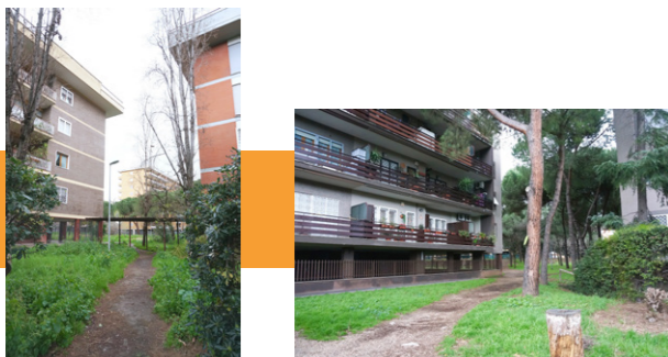
Figure 2.17. Tertiary Street Photos
