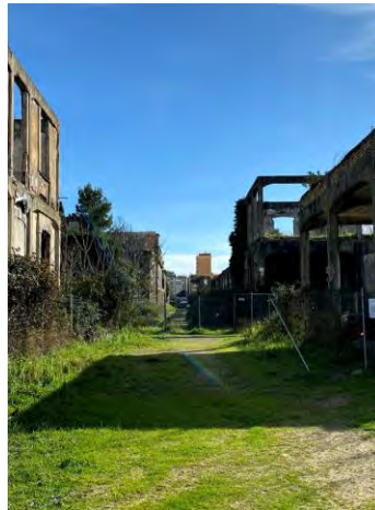
Figures 52: Photo of Abandoned Factory
