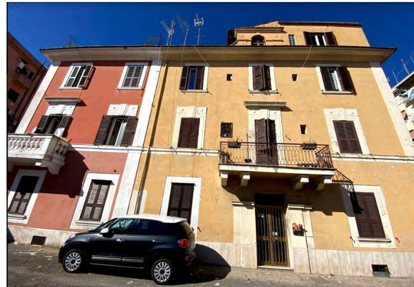
Figure 32: Photo of Villini on Via Pausania
