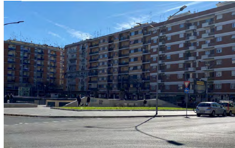
Figure 31: Photo of Intensivi surrounding Piazza Malatesta
