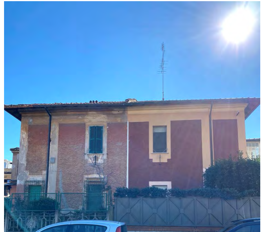
Figure 56: Photo of Housing in Garden City, Prenestino
